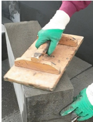
Grinding FOAMGLAS®
