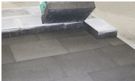
Staggered joints between FOAMGLAS® layers
