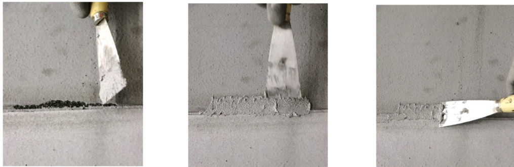
Repair of the FOAMGLAS® INVATHERM™ coating
