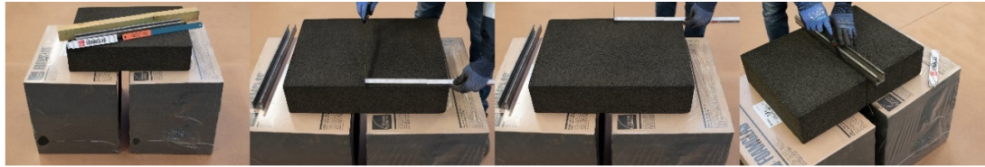
Preparation for cutting FOAMGLAS®
