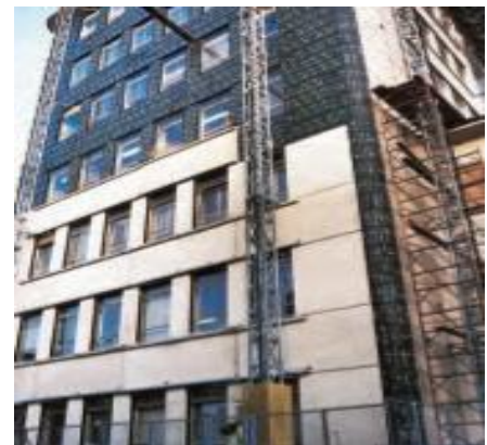
FOAMGLAS® insulated facade
