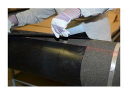
**Step 5**Apply pressure to ensure that jacket achieves adhesion without trapping air.
