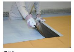
**Step 3**Slit the release film at this overlap, taking care not to slit jacket. Remove release film except at the overlap. Dirt and dust must be kept off jacketing.
