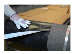
**Step 6**Remove the remaining release film on the overlap and press tightly to seal the longitudinal joint.
