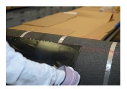
**Step 4**Starting on the chalk line, press the surface of the jacketing halfway around the FOAMGLAS® insulation. Best results are achieved when the starting point results in the overlap terminating in a water shedding position.
