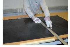
**Step 2**Cut a section of jacketing long enough to fit around the insulated pipe and have a 2 in. (50 mm) overlap.
