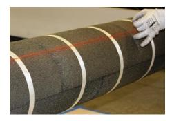
**Step 1**After FOAMGLAS® insulation is installed, strike a horizontal line along the insulation convenient for starting jacket positioning and to ensure a uniform lap line.
