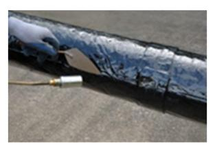
NOTE: The lap is closed with opening facing upward to allow softened bitumen to flow into open seam. This provides a positive seal. This technique is the opposite of conventional jacketing applications.
