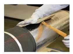
**Step 6**Remove the remaining release paper on the overlap and press tightly to seal the longitudinal joint.
