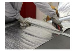
**Step 2**Cut a length of jacketing to provide at least a 2 in. (50 mm) overlap at the longitudinal seam.
