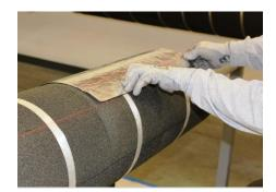
**Step 4**Starting on the chalk line, press the surface of the jacketing halfway around the FOAMGLAS® insulation.
