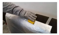
**Step 4**Apply pressure with plastic spreader to ensure that the butyl adhesive fills the surface cells of the insulation and achieves adhesion without trapping air.
