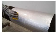
**Step 7**Apply pressure with spreader to ensure that the jacketing overlap is well adhered and without air bubbles. This completes installation of one section of jacketing.
