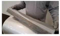
**Step 2**Peel 2 in (50 mm) of release film from the jacketing to reveal the butyl adhesive.
