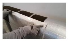
**Step 9**Continue applying jacketing sections as described above, taking care to overlap and offset the starting point of each section from the previous one.
