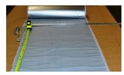
**Step 1**Cut a section of jacketing long enough to fit around the insulated pipe and have a 2 in (50 mm) overlap.
