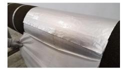
**Step 6**Remove remaining release film and press jacketing around the circumference to achieve adhesion without trapping air.
