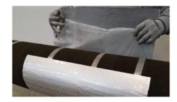
**Step 5**Remove release film while applying jacketing around the circumference of the insulation.
