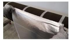
Apply revealed adhesive to insulation in line with pipe axis. Best results are achieved when the start point results in the overlap terminating in a water shedding position.
