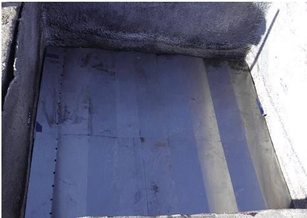
Figure 14: FOAMGLAS® PFS System (Gen 2), placement in the LNG pit
