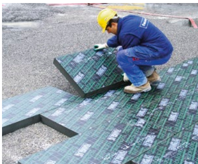
Pannelli FOAMGLAS® Boards, applicati a secco
