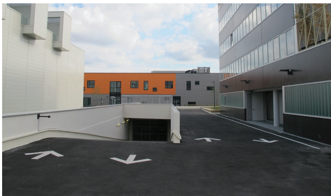
Parking Zac des Louvresses, FR - Gennevilliers
