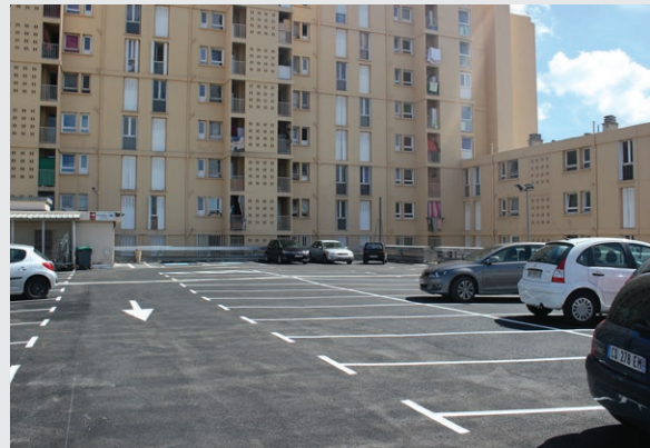
Renovatie parking Carrefour Market Plombières, FR - Marseille
