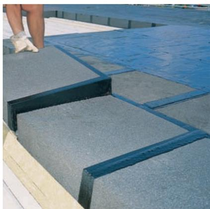
The Kalzip FOAMGLAS® System is ideal for projects where the moisture and temperature conditions place particularly challenging demands regarding vapour-control and permanent risks of condensation to form. The system is also ideal for sensitive production areas, e.g. clean rooms for producing or storing electronic components, where a perfectly sealed building envelope is essential.
