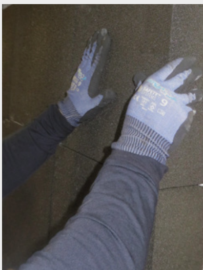
Pose de FOAMGLAS®
