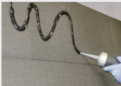
Application du coating
