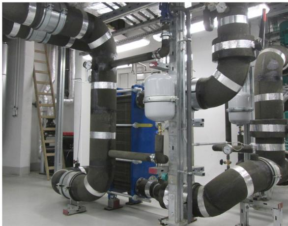
Chilled water systems are frequently installed in large buildings, stadiums or facilities, where fire safety is always a key requirement. Because FOAMGLAS® insulation is 100% glass, without binders or fillers, it will not burn, even when in direct contact with intense flame.
