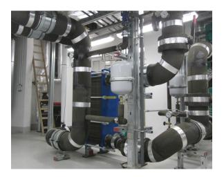
Chilled water systems are frequently installed in large buildings, stadiums or facilities, where fire safety is always a key requirement. Because FOAMGLAS<sup>®</sup> insulation is 100% glass, without binders or fillers, it will not burn, even when in direct contact with intense flame.
