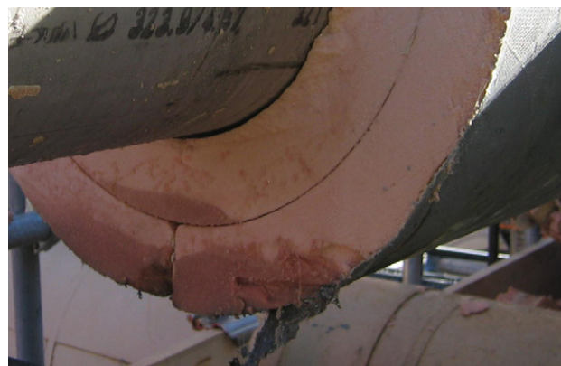
Moisture accumulation in PU foam system due to breach in vapor barrier.
