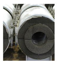
FOAMGLAS® insulation is most suited to use in "dead weight load" support applications where the pipe is resting in a band style hanger, or on a rolled plate cradle. It is not suited for use in guides, (spider or cryogenic service) where thermal forces (live loads) can be in a magnitude much greater than simple dead weight load.
