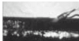
11 Burn off polyester film for distance of 2" back at butt lap seal.
