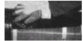
4 Starting on the chalk line, press PITWRAP® jacketing half way around FOAMGLAS® Insulation.
