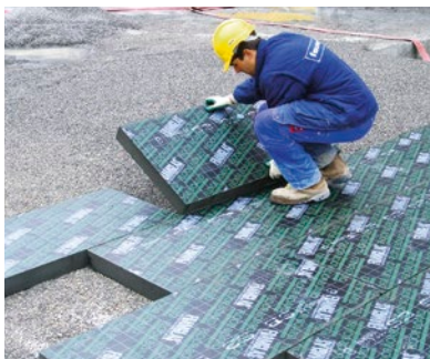
Pannelli FOAMGLAS® Boards, applicati a secco
