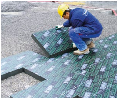
FOAMGLAS® Boards in Trockenbauweise
