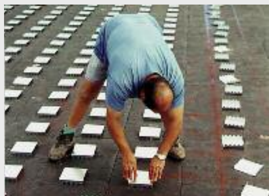
FOAMGLAS® insulation structures do not require any mechanically penetrating fastening devices to take up the covering. The sheet metal covering is assembled with "claw plates" (PC® fixing plates).
