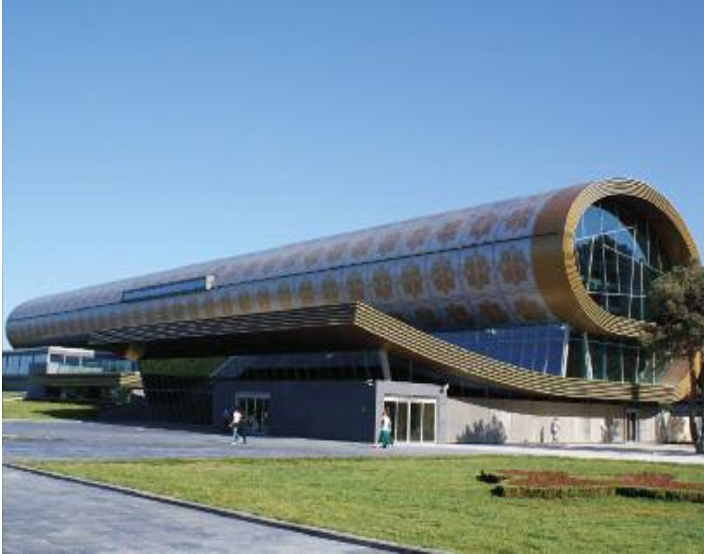
Metal façade and roof
