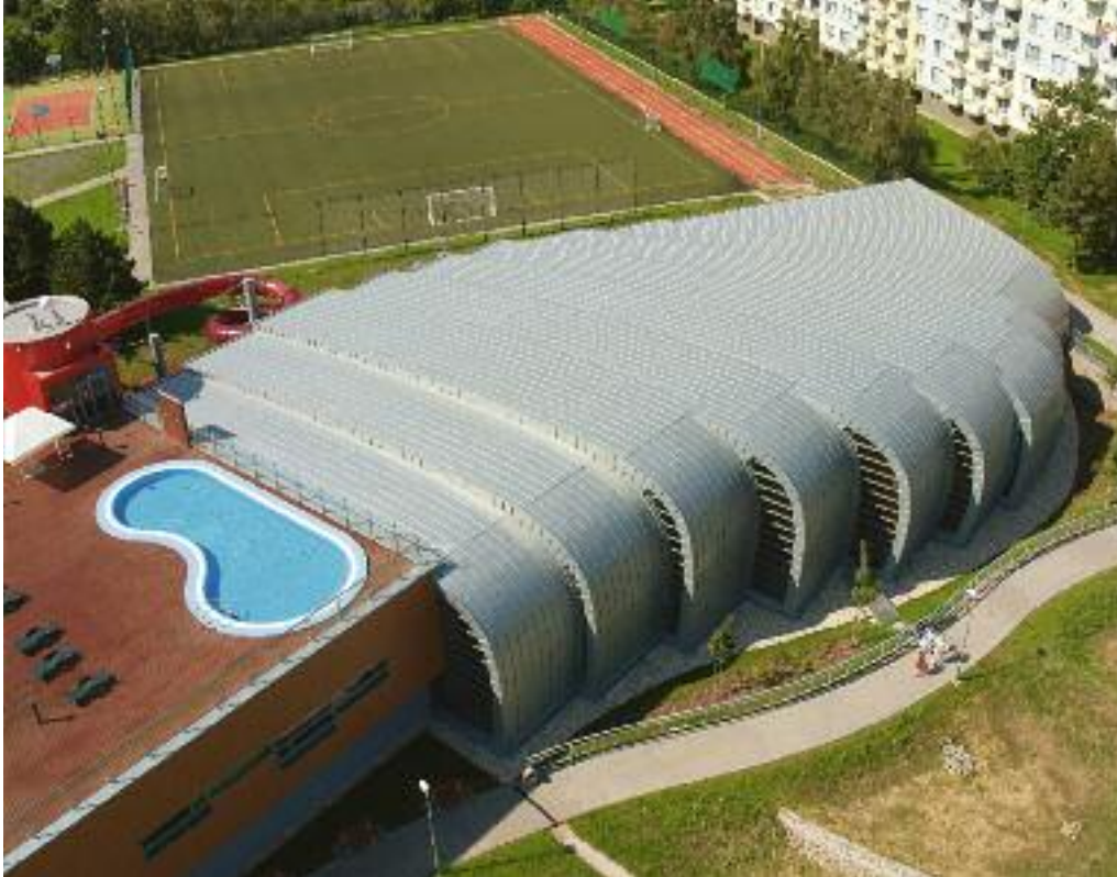
Metal standing seam roof over aqua-park
