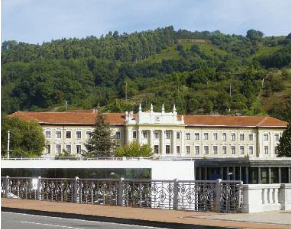
Pitched roof with tiles
