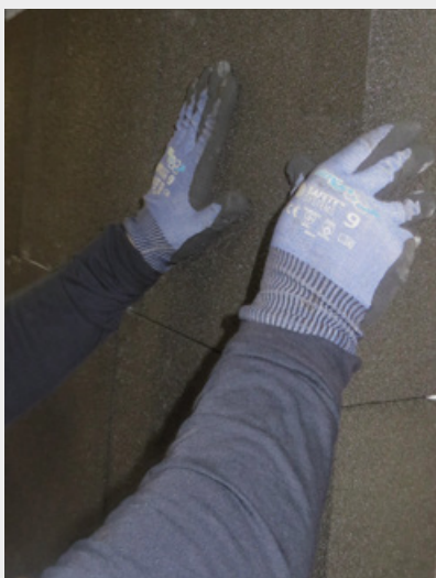
Pose de FOAMGLAS®
