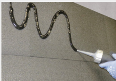
Application du coating
