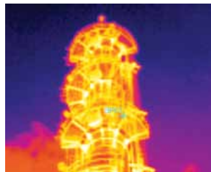
Thermal imaging can identify hidden problems.
