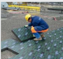
FOAMGLAS® FLOOR BOARD posato a secco
