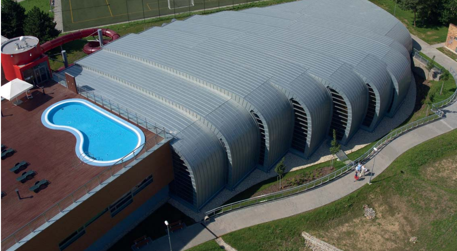
Aquapark, Brno – Kohoutovice, Czech Republik – Architect Atelier K4
