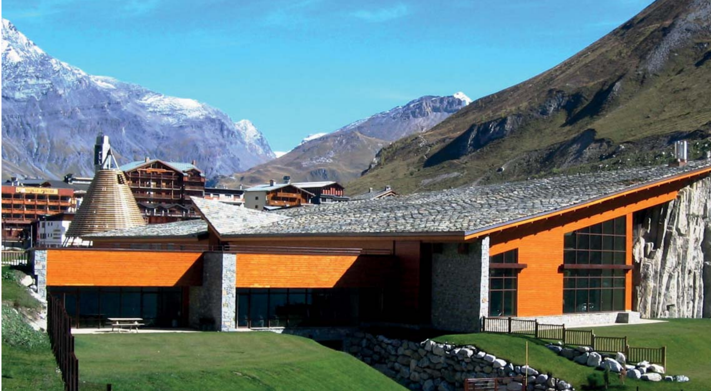
Le Lagon aquatic area, Tignes – DHA architects
