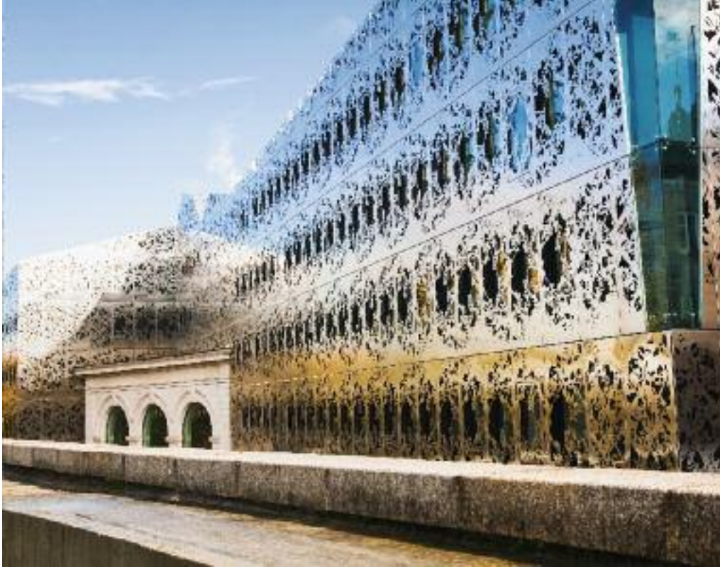
Perforated cladding, stainless steel façade cassettes
