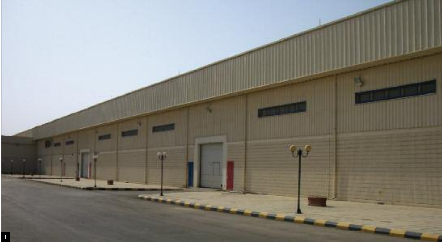
1 Industrial building, cold store.
