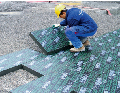
FOAMGLAS® Boards in Trockenbauweise
