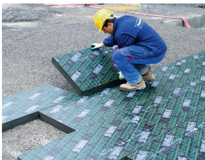
Pannelli FOAMGLAS® Boards, applicati a secco
