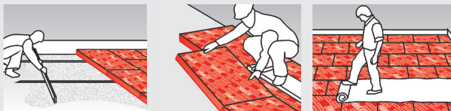
Pannelli FOAMGLAS® Boards, applicati a secco
