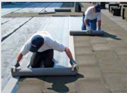
Pose des plaques FOAMGLAS® T3+, T4+, S3, F
