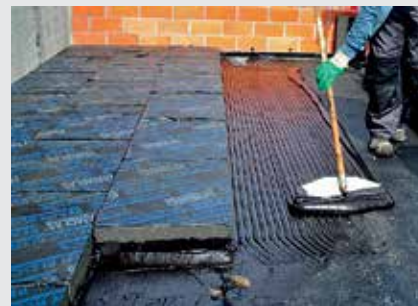
Pose des panneaux FOAMGLAS® READY BLOCK T3+, T4+, S3, F
