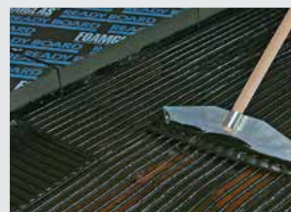
Pose des panneaux FOAMGLAS® READY BLOCK
