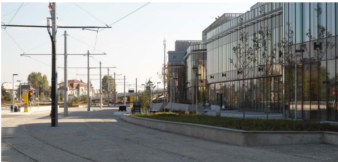
Roofs accessible by trucks and trams Gallery Šantovka, Olomouc, Czech Republic
