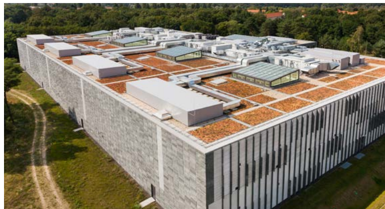
Technological roofs Metroalde, Bilbao, Spain
