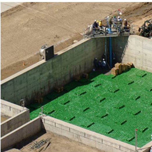
THE FOAMGLAS® PFS GEN 1 SYSTEM INSTALLED AT LNG FACILITY IN THE US
