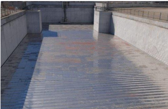
THE FOAMGLAS® PFS GEN 2 SYSTEM INSTALLED AT AN LNG TERMINAL IN THE US
